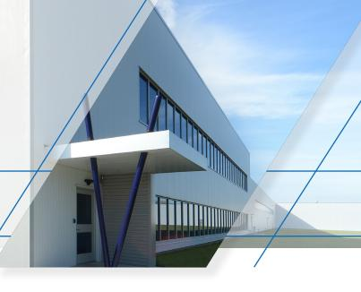
The Metl-Span CF Mesa insulated metal panel is well suited for exterior and interior walls and ceiling applications. The lightly corrugated profile on both faces creates symmetry on the outside of the building and room to room within. The minor rib provides a flattened appearance. Mesa panels are ideal for commercial, institutional and industrial applications.
